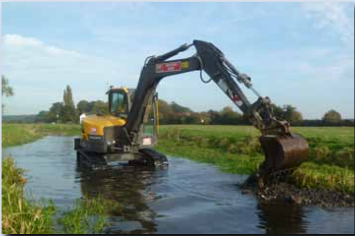
River restoration at Seaton used excavators to dig pools in the river and re-engineer the banks to benefit local wildlife
