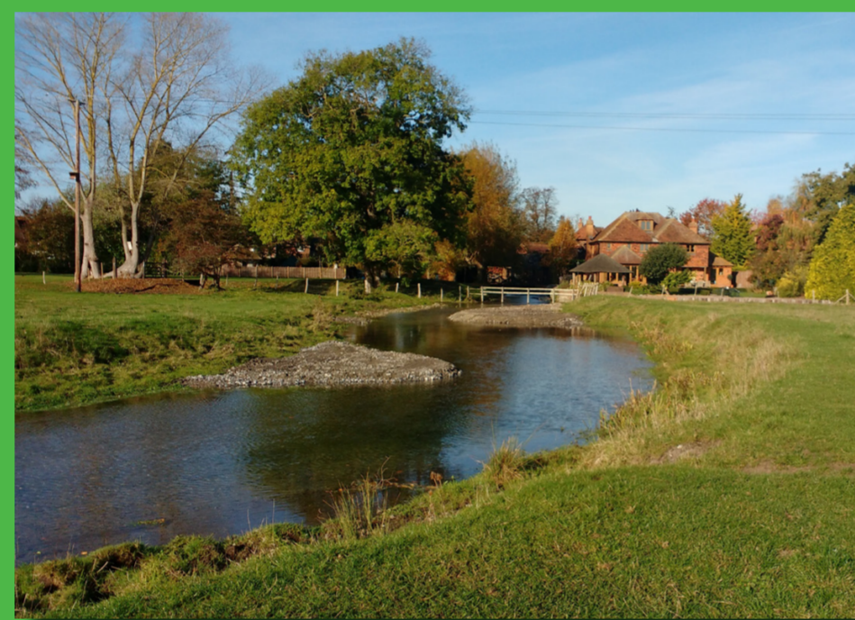
Newly created 'berms' in the Little Stour create a more natural, meandering shape
