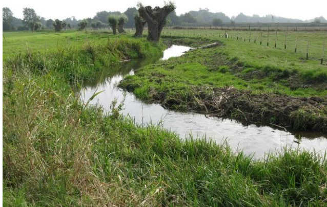
At Godinton the channel has been narrowed by using faggots to create a faster flowing channel.
