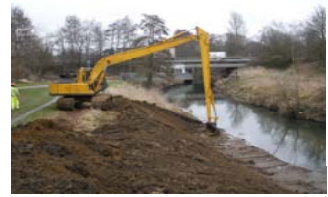
Before and during works
