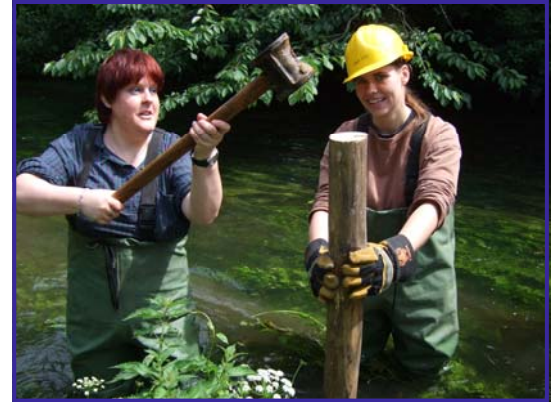
Carrying out bank protection work in Chartham
