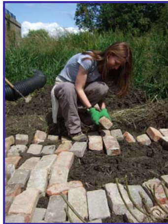
Working on the otter holt, Canterbury
