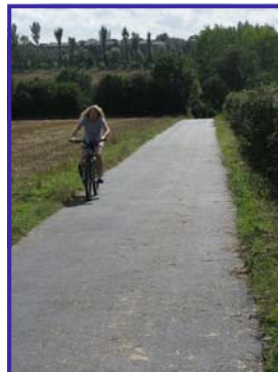
Tarmacing completed near Blean church on the Crab & Winkle Way
