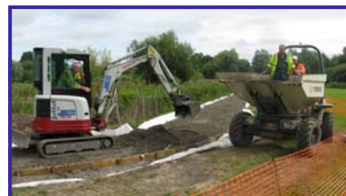
Construction of the Canterbury to Chartham shared use path
