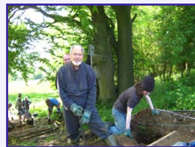
Installing steps at Cherry Downs
