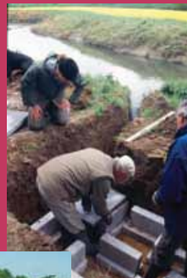
Otter hole construction
