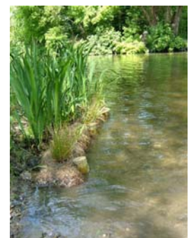
Fig. 29 Example of coir rolls
